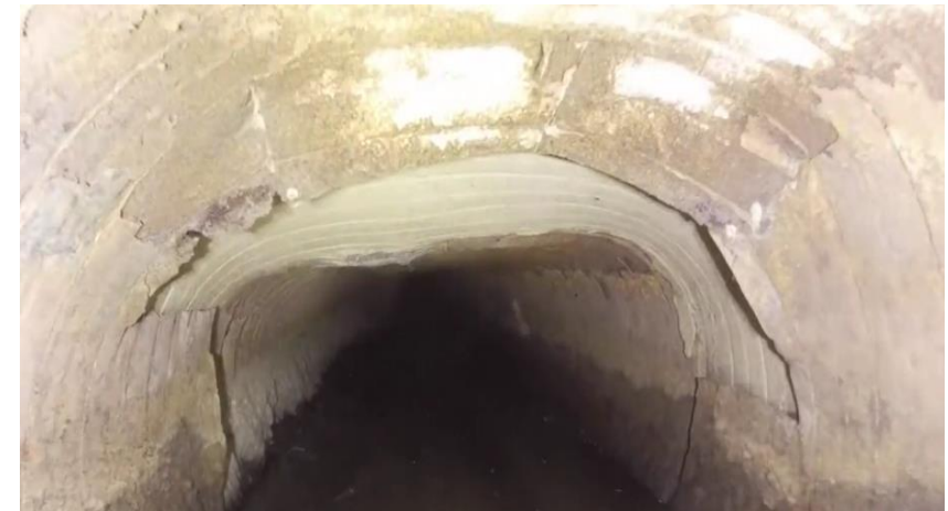
Canal Internal Inspection
