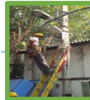
Lineman attending complaint (Self Supervised)
